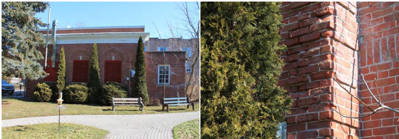
Figures 58 & 59: (left) View of west elevation, looking east (right) Detail view of south corner of west elevation noting damages to masonry (Source: MHBC, 2018)
