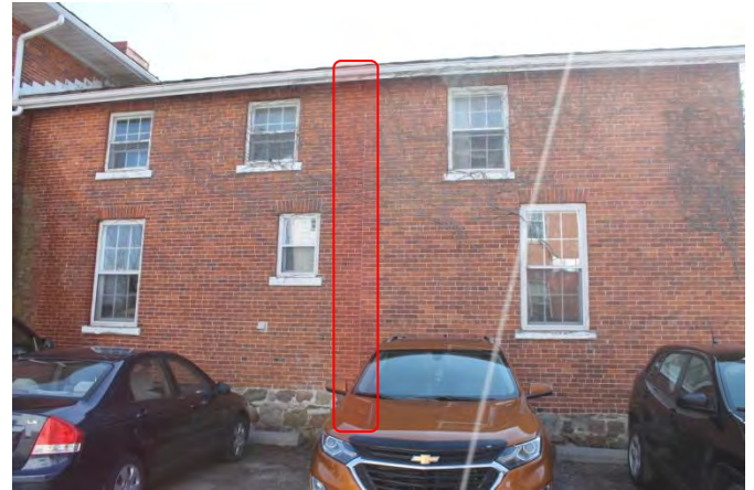
Figures 43 & 44: (left) View of north elevation, looking south (right) Detail view of north elevation, looking south. Red box notes location of division line between first and second brick additions (Source: MHBC, 2018)
