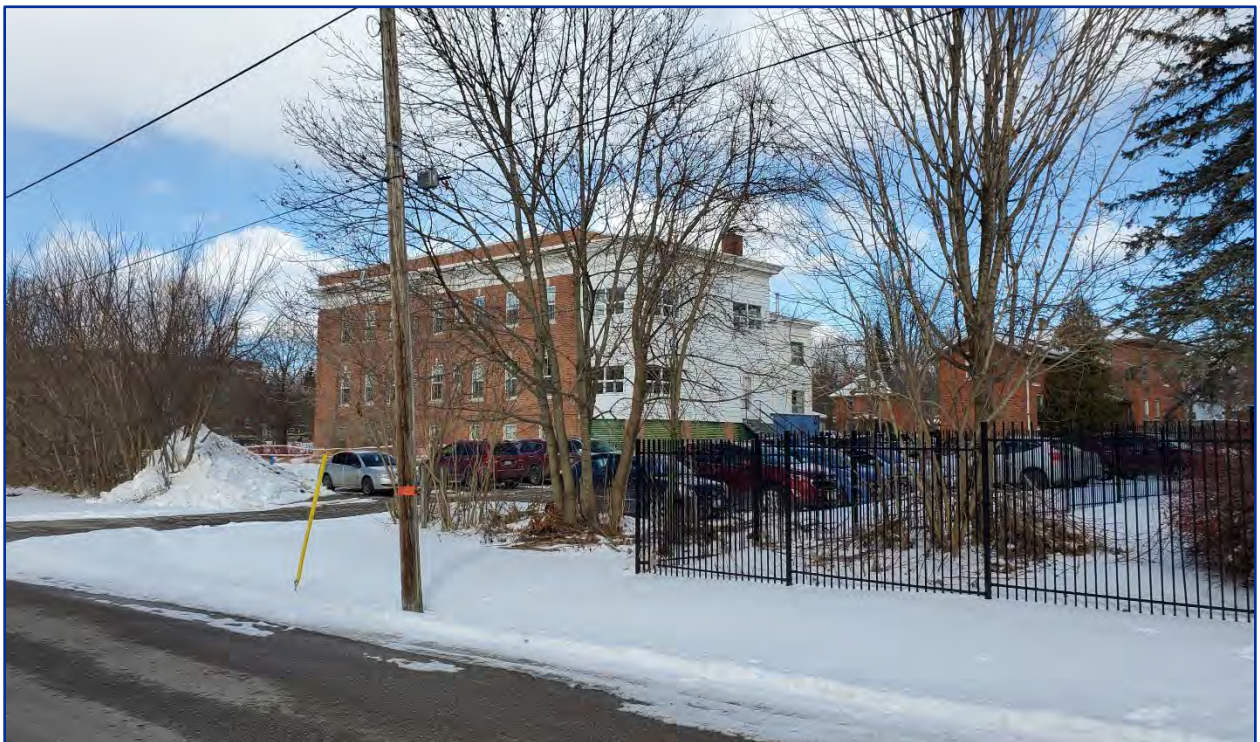
Figure 4: View north of southwest corner
