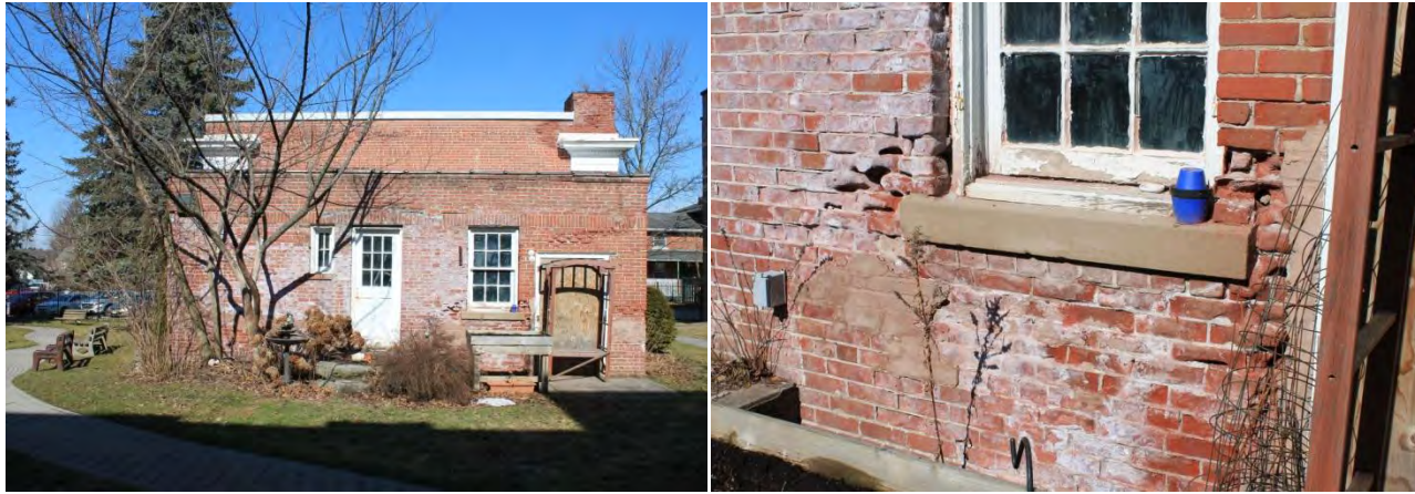
Figures 56 & 57: (left) View of south elevation, looking north (right) Detail view of bricks at south elevation noting damage to masonry (Source: MHBC, 2018)
