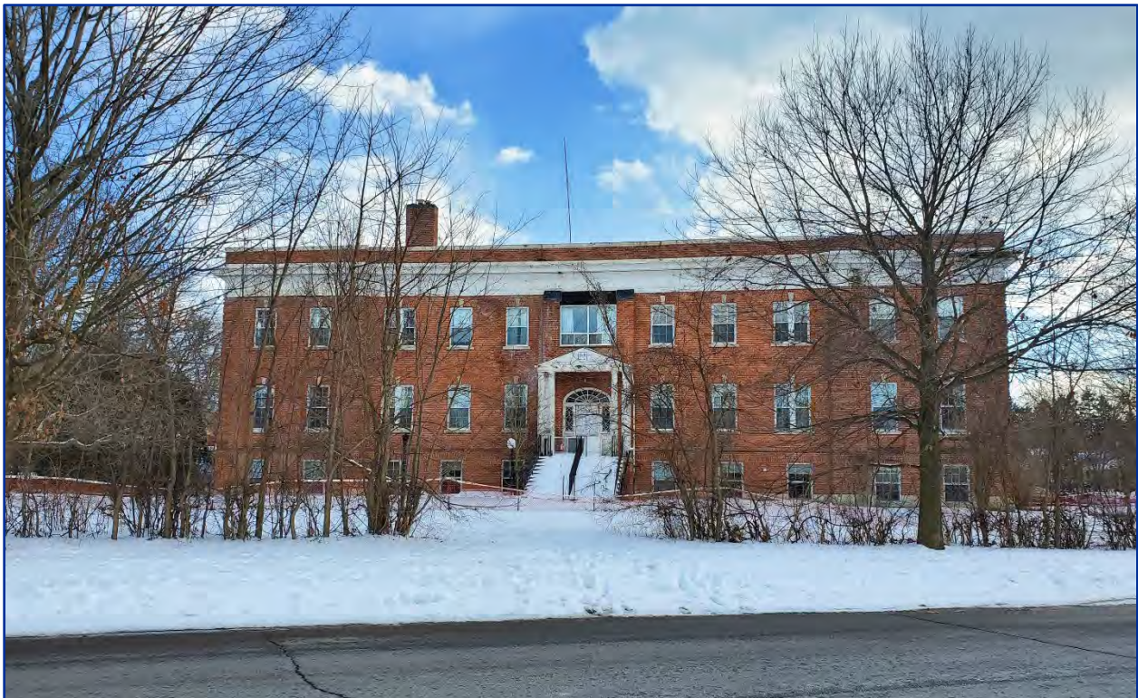
Figure 2: View south of north elevation
