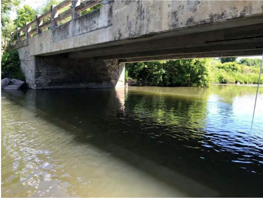
Photograph 7 – Sylvan Glen Bridge looking northeast – June 14, 2022
