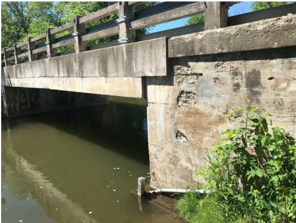
Photograph 8 – Sylvan Glen Bridge span looking southwest – June 14, 2022
