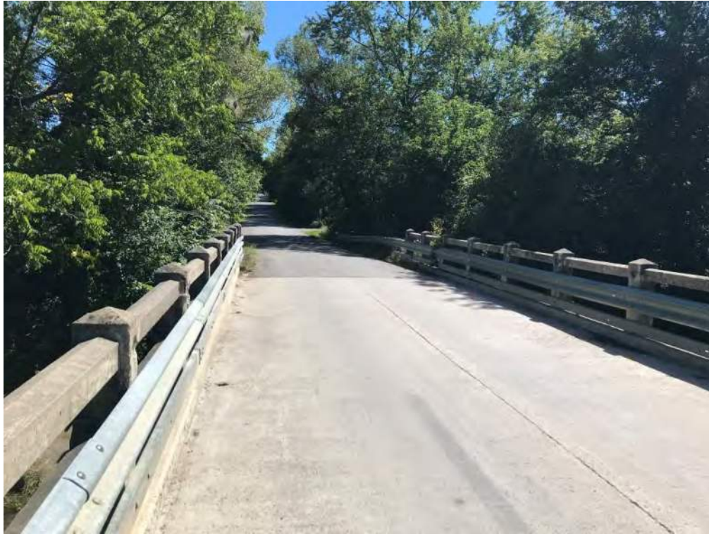
Photograph 5 – Sylvan Glen Bridge – Facing South – September 1, 2022
