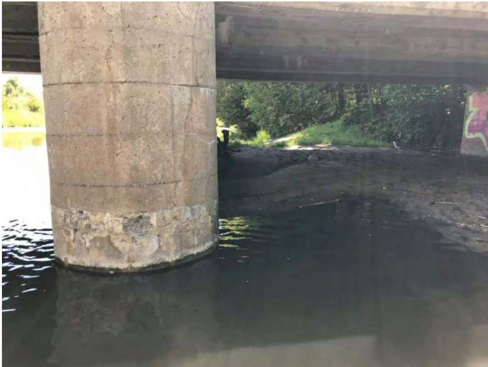
Photograph 6 – Sylvan Glen Bridge pillar southwest side of the bridge – June 14, 2022
