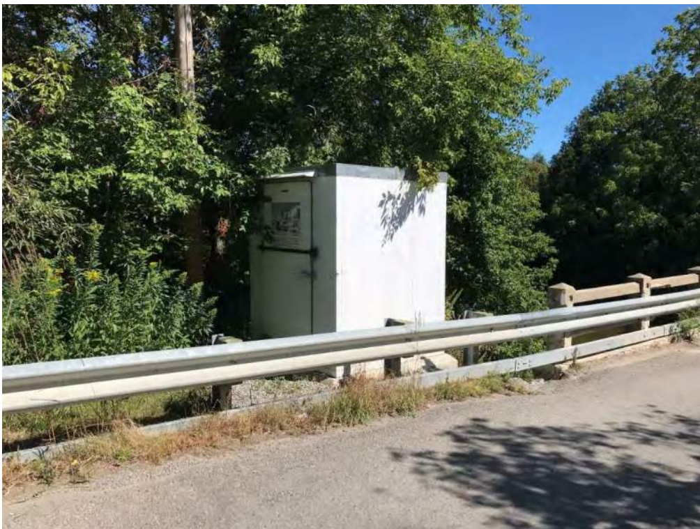
Photograph 4 – Environment Canada Monitoring Station and single utility pole located northeast of the Bridge - September 1, 2022
