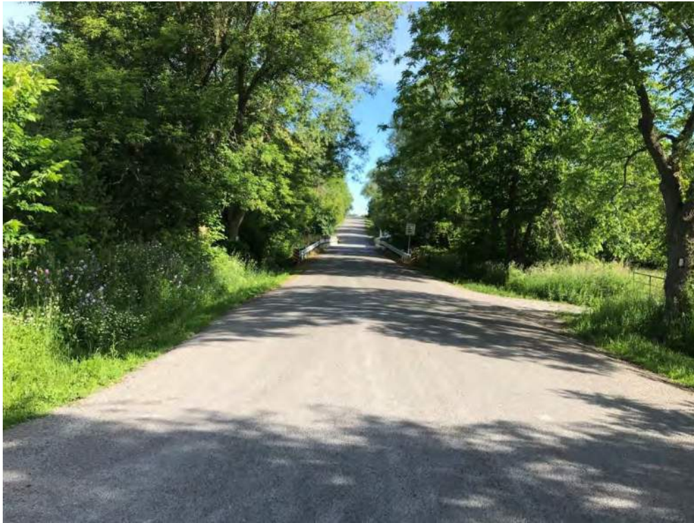
Photograph 1 – Sylvan Glen Bridge – Facing North – June 14, 2022
