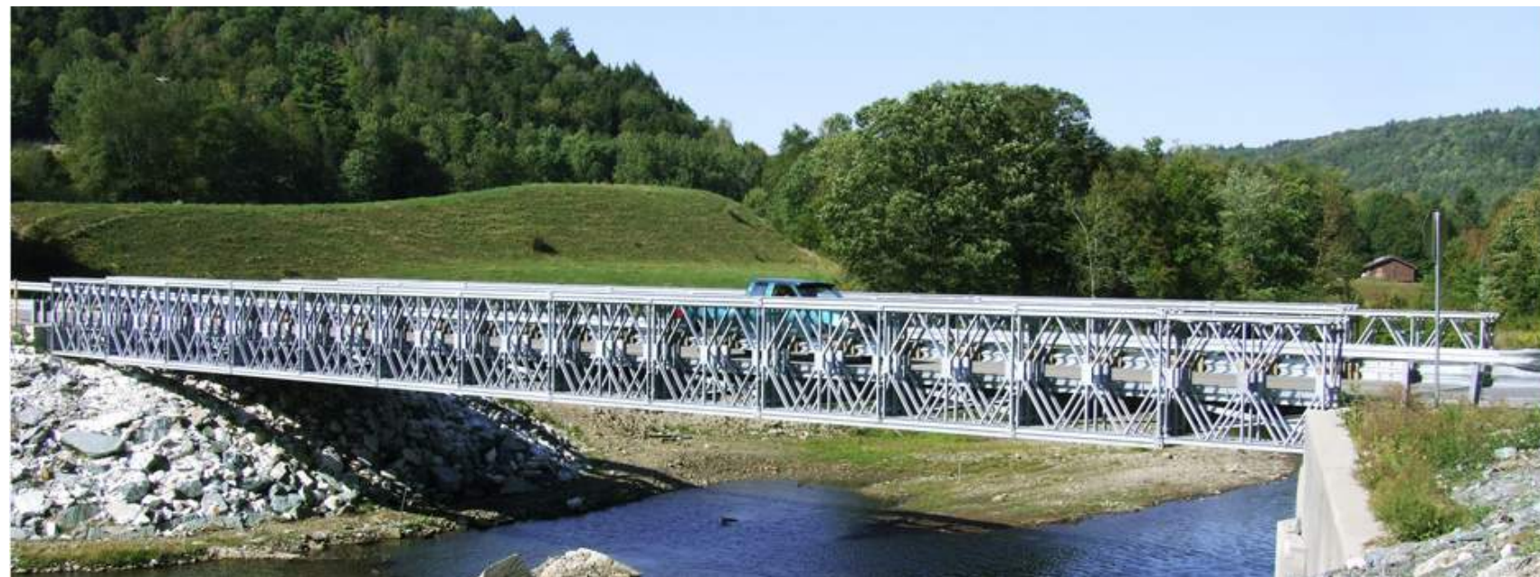
Modular Steel Panel Bridge Example
