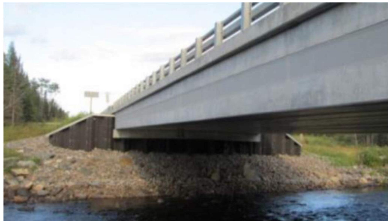
Semi-integral Bridge Example
