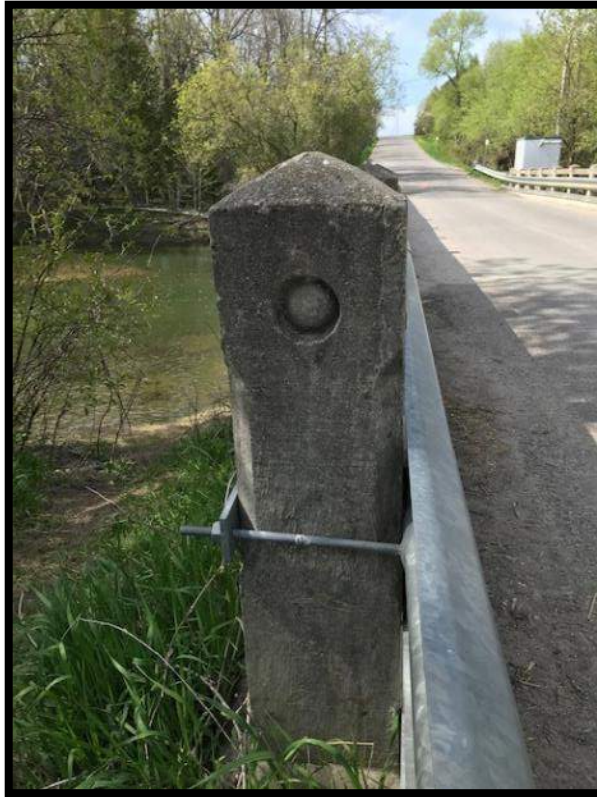
IMAGE C - Chamfered Post Detail (Ainley Group 2022)
