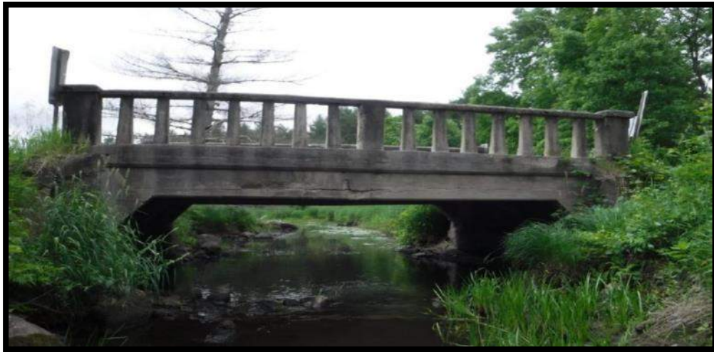
IMAGE E1 - Greatrix Bridge - Municipality of Tweed built 1925 (Greenview Environmental 2018)
