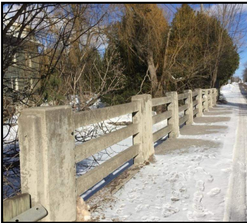
IMAGE E2 - Westwood Bridge - Westwood, County of Peterborough built 1937 (Ainley Group 2018) (prior to recent demolition and reconstruction)
