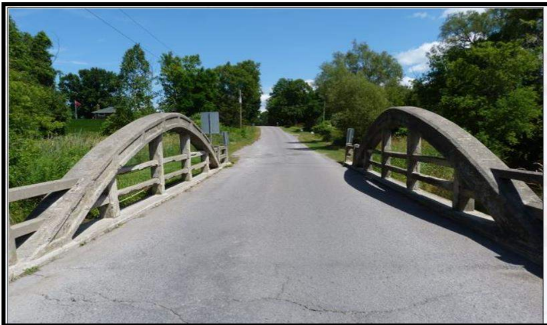
IMAGE E4 - Sackville Bridge - Cavan Road, Northumberland County built 1920s (Nathan Holth – www.historicbridges.org )
