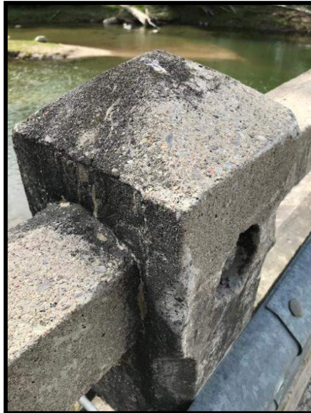
IMAGE B – Chamfered Post & Rail Insertion (Ainley Group 2022)
